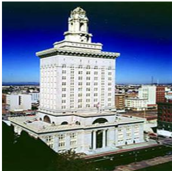
Fig. 7 Oakland City Hall
